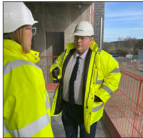
Visiting the site of the new HMP Highland in Inverness which will house prisoners from across the region.
